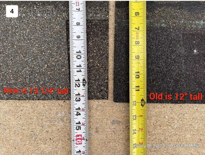
Closer view of the overall height between the discontinued shingle and the current shingle.
