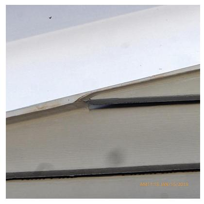
This lower photo is an example of the loose edge of the tops of many planks along the roof fascia.
