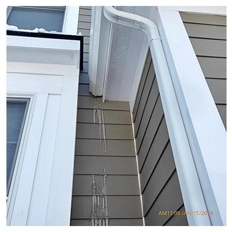
Water has been dripping where the garage wall abuts the main house. Ice has formed obviously. A length of sheet metal has been installed to deflect water from hitting the box window trim, but there was deep snow and it could not be determined if kick-out flashing is present against the house. The gutter is close to the siding, but it was not measured, but JH recommends an inch from the siding.
