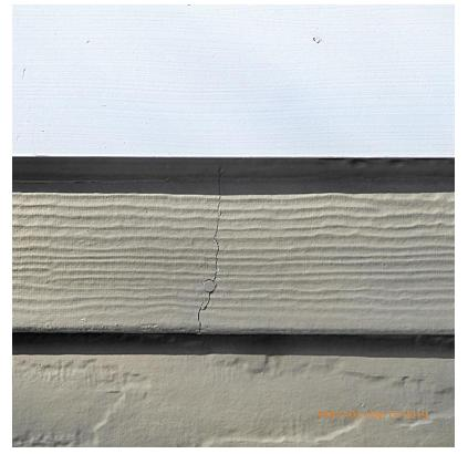
The nail here was driven so hard it cracked the siding under this window trim.
