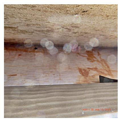
When this very loose plank was lifted water marks could be seen.
