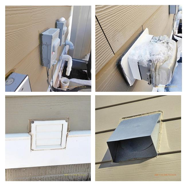
These are other examples of various penetrations not placed on a proper mount, or installed directly into the siding.
