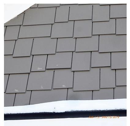
The shingles on the front of the house, over the garage door, were all wavy, erratically placed where edges did not make sense, and had touch-up paint over face nails that did not match.
