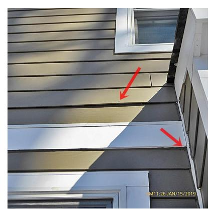
More examples of poorly installed siding and trim.
