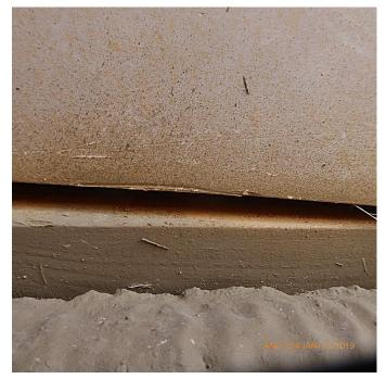
Looking under the box penetration housing the fireplace it could be seen that the gap between the soffit cover and the sides and where it abuts the house was never caulked.
